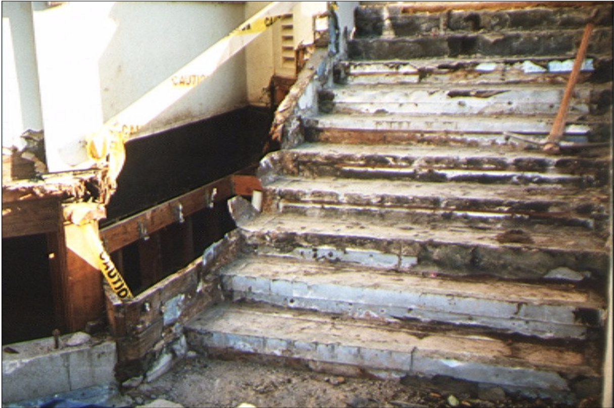
Kitchen Stair & Planter Testing
