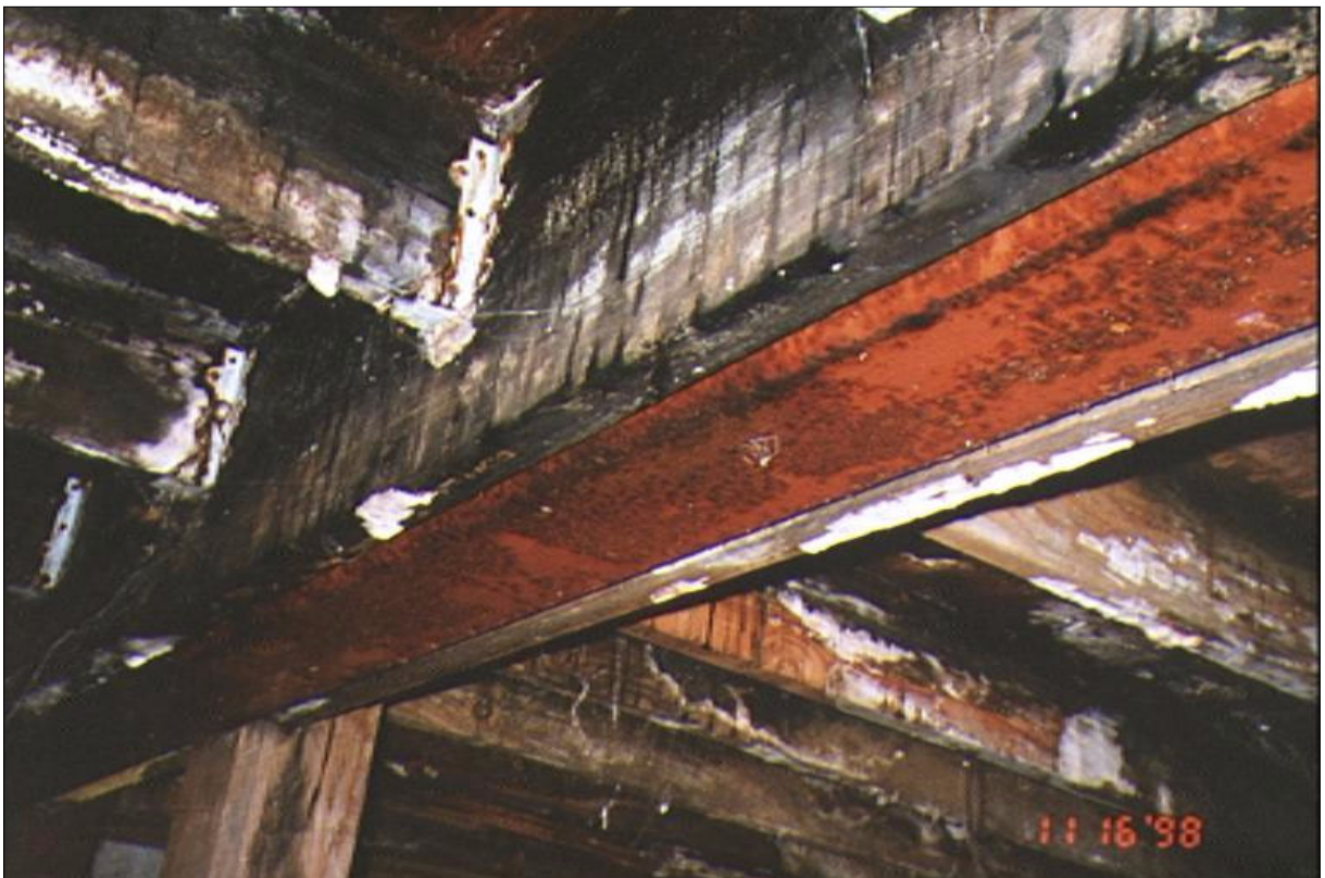
Central Deck Frame & Steel
