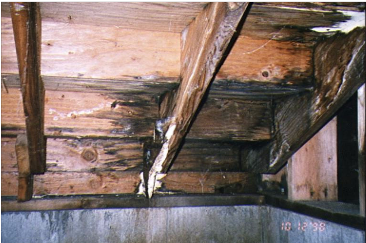
Kitchen Deck Stair Underside
