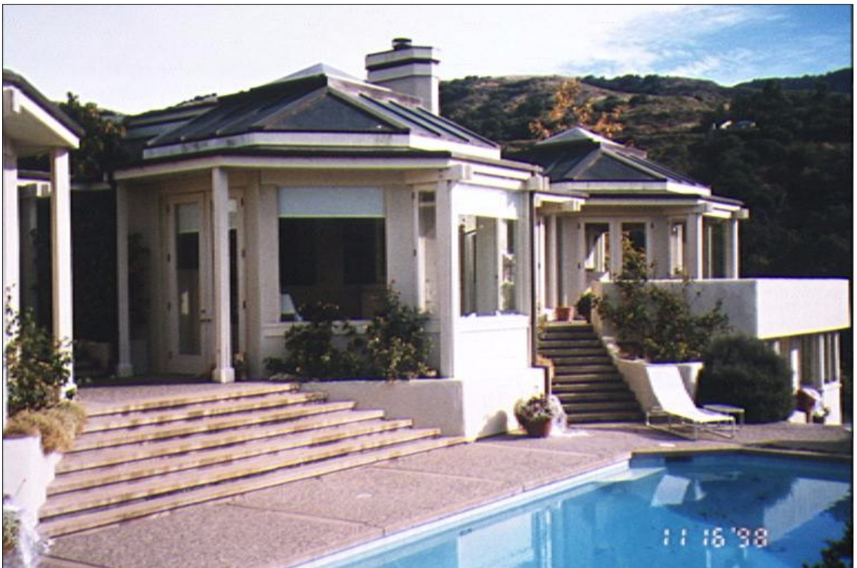
Central Deck & Kitchen Stair (Right)
