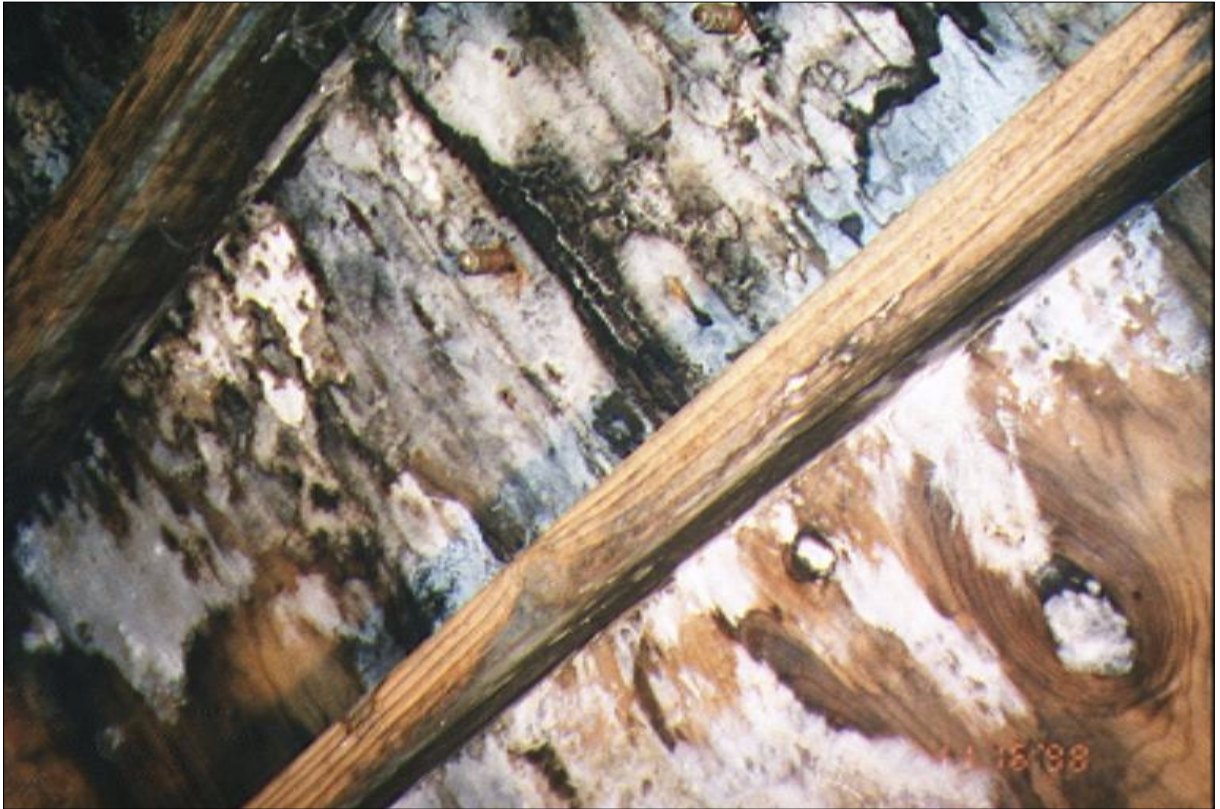
Central Deck Underside - View 2
