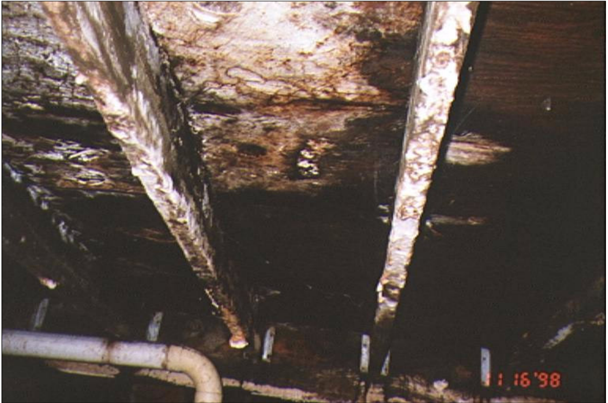
Central Deck Underside
