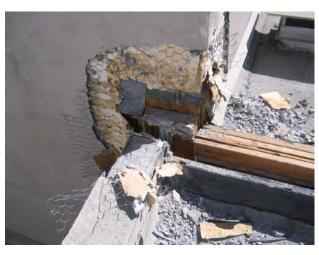
Removing stucco to investigate waterproofing layers underneath to determine the source of the leaks.
