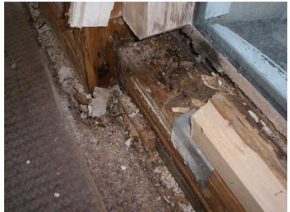
MFC designed a costeffective way to replace the windows that had leaked and repair the damage.
